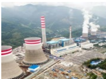
The 1,320-megawatt Chongqing Songzao power plant in Chongqing, China
